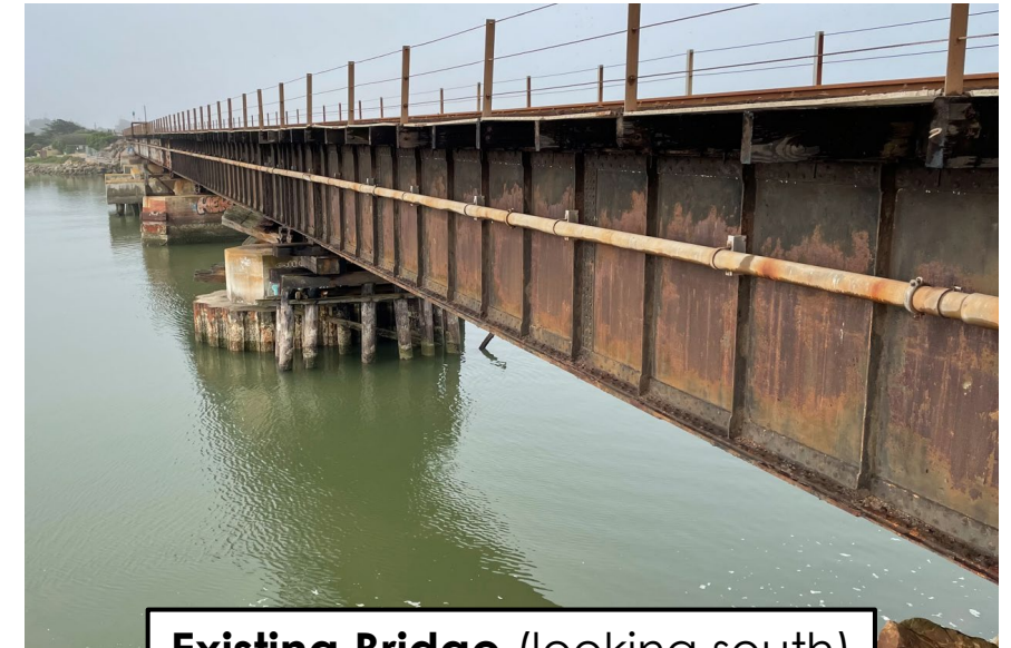
Existing Bridge (looking south)
