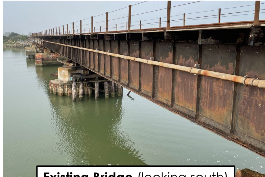
Existing Bridge (looking south)
