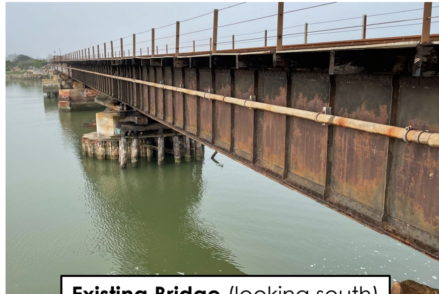
Existing Bridge (looking south)
