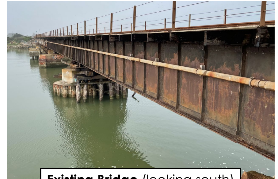
Existing Bridge (looking south)
