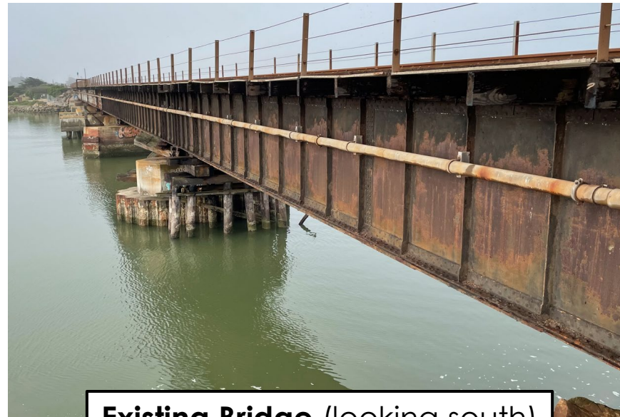
Existing Bridge (looking south)
